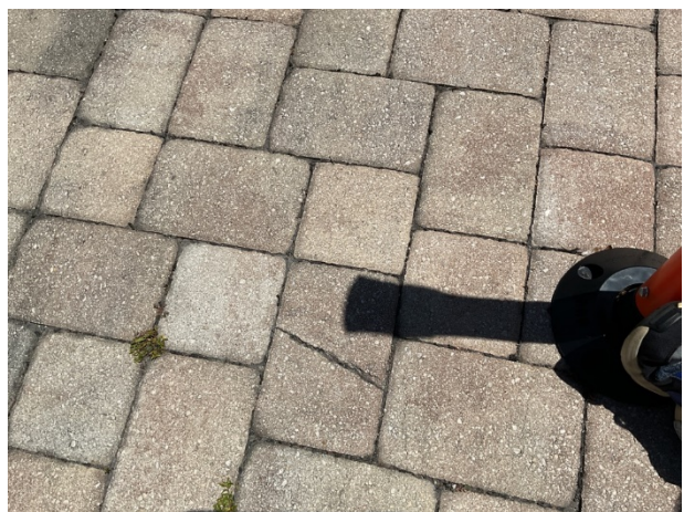
Pavers cracks
