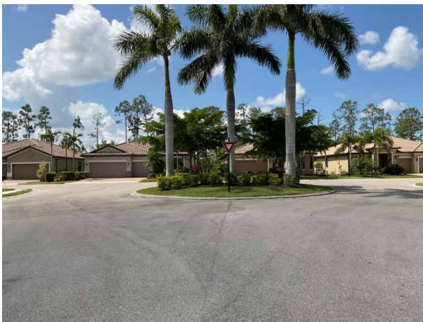
Asphalt pavement street overview
