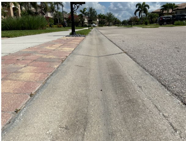
Concrete gutter overview
