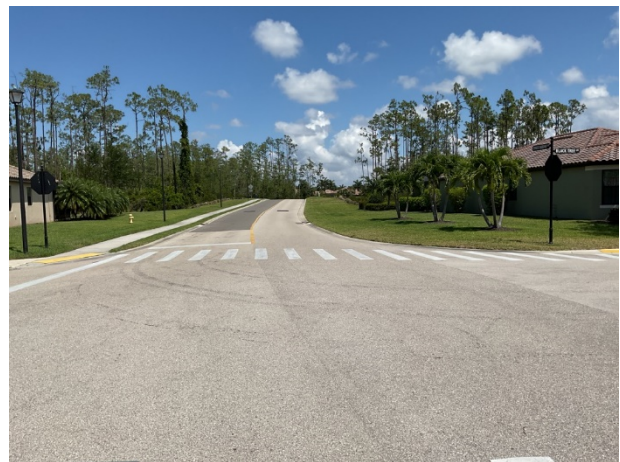
Asphalt pavement street overview
