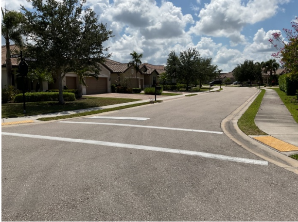
Asphalt pavement street overview
