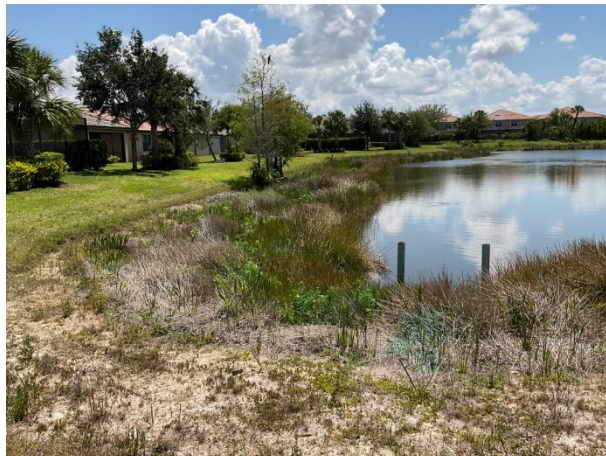
Minor shoreline erosion remediation
