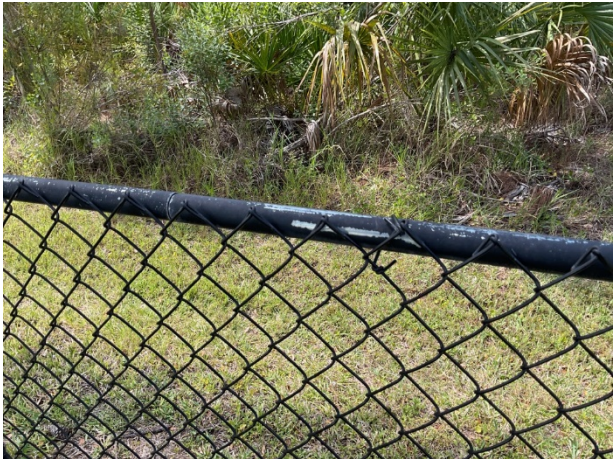
Finish deterioration
