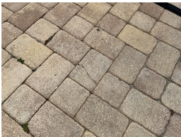
Paver cracks
