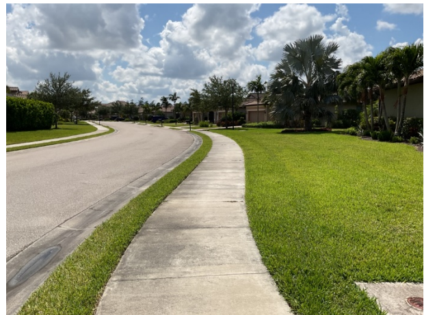
Concrete sidewalk overview
