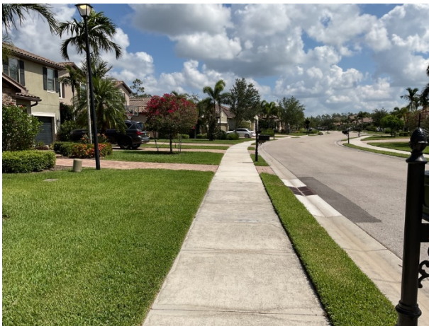
Concrete sidewalk overview
