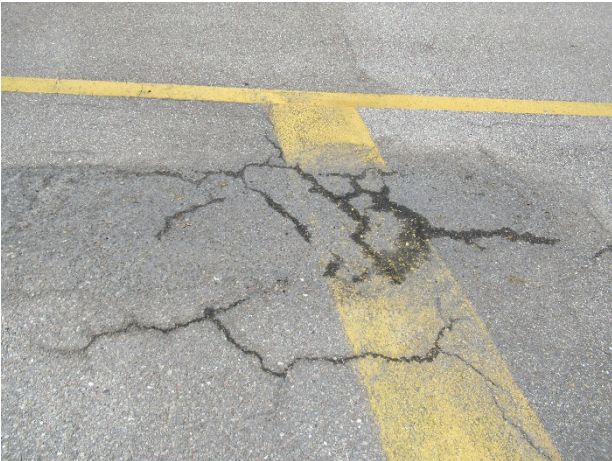
Pavement cracks
