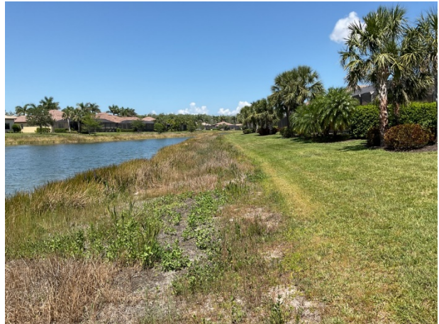
Minor shoreline erosion remediation
