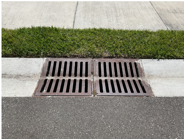
Catch basin overview
