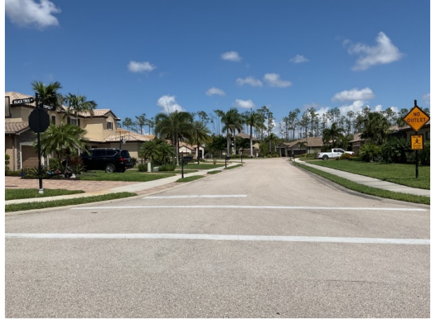
Asphalt pavement street overview
