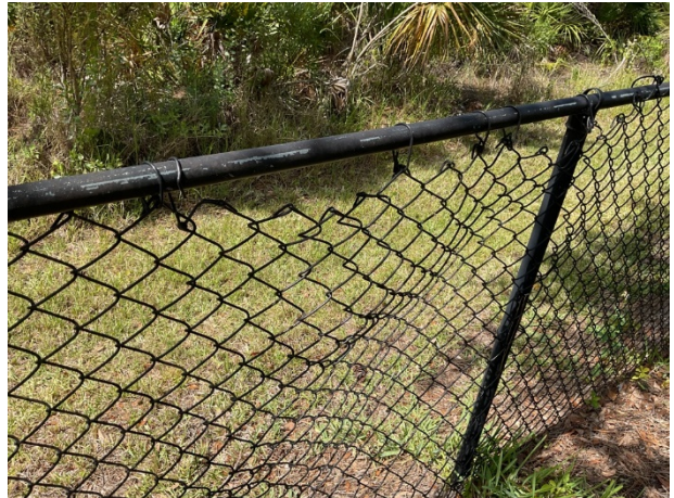
Fence warped webbing
