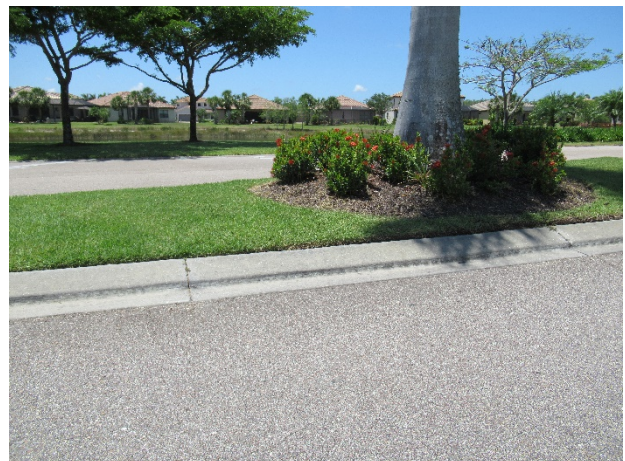
Concrete curb overview
